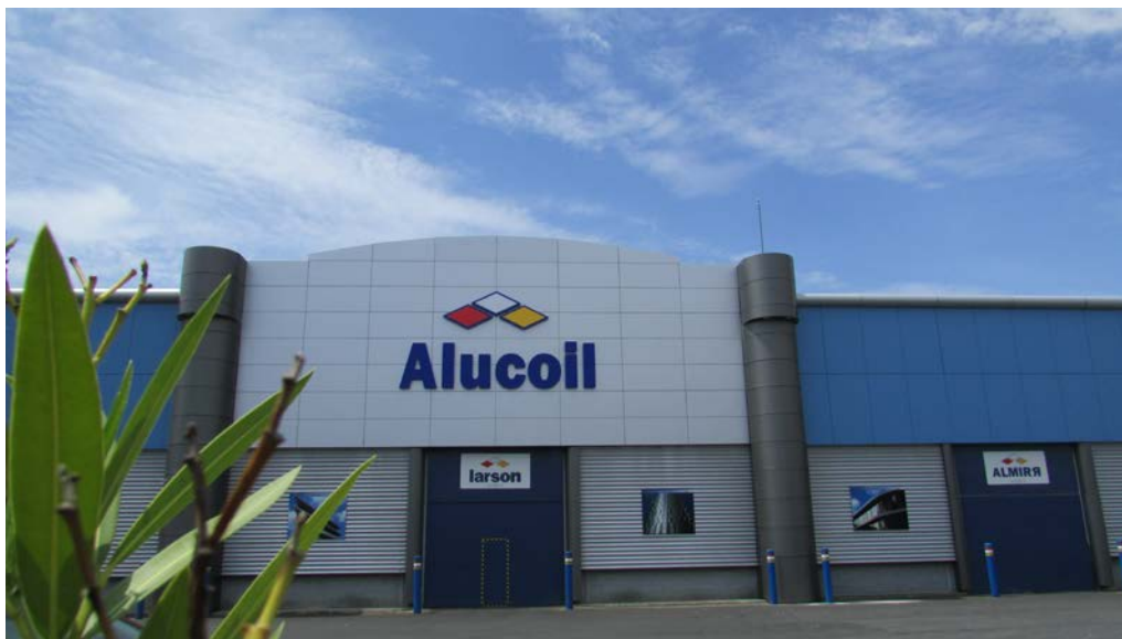
Picture 1: Installations of Alucoil, S.A. in Miranda de Ebro. Source: ALUCOIL S.A.
